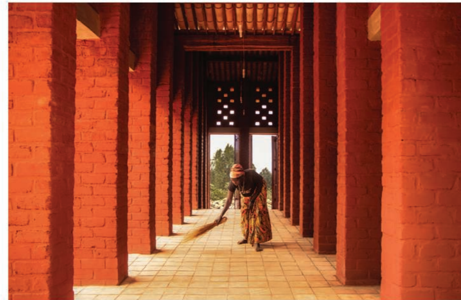
view of entrance and external hallway
